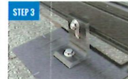
ATTACH L-FOOT TO RAIL
