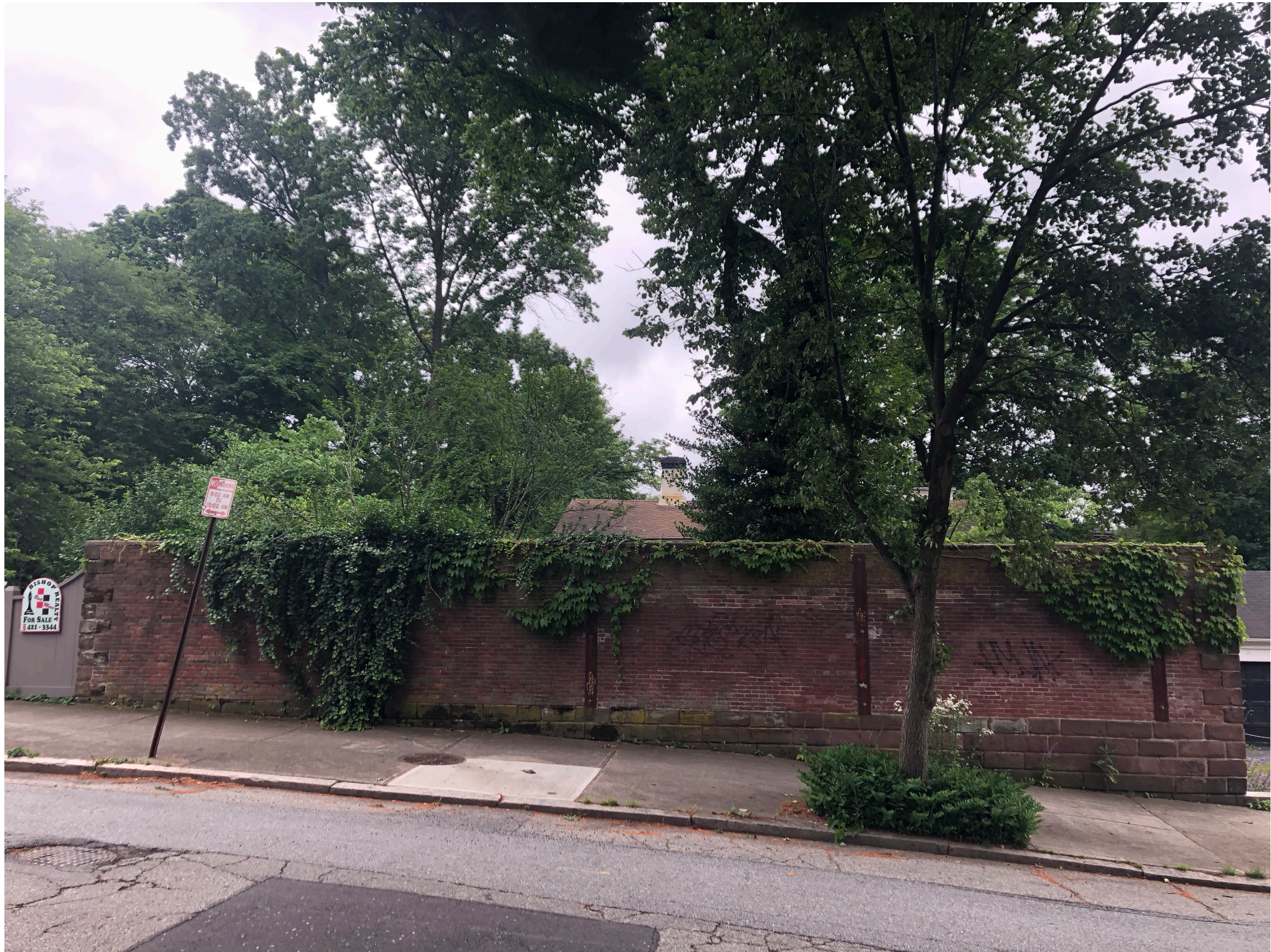
59 WILLIAMS STREET EXISTING BROWNSTONE & BRICK WALL
