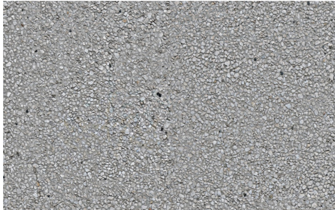
Exposed Aggregate Concrete Base
