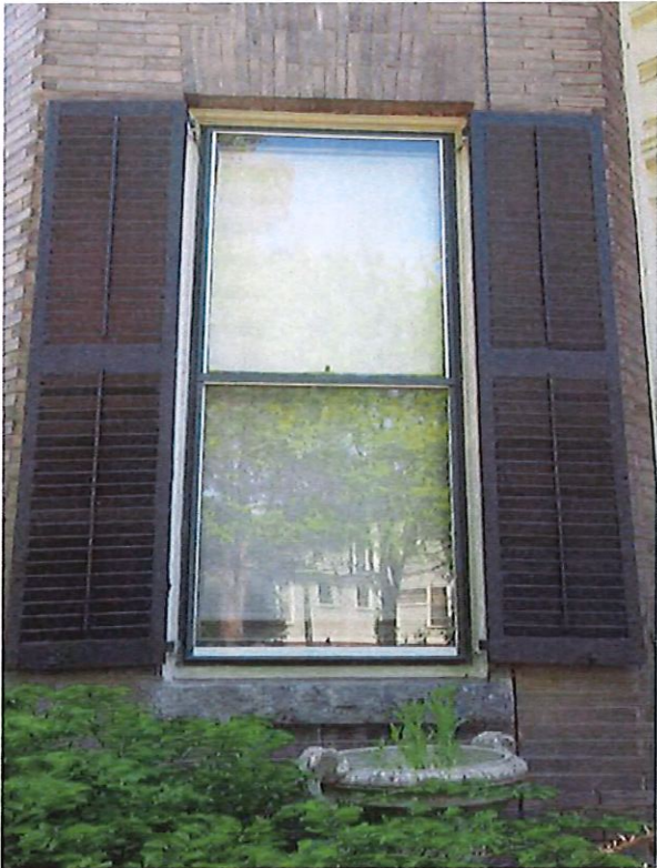
FIGURE 5: North Elevation (First Floor Window)
