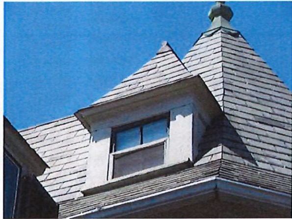
FIGURE 6: North Elevation (Third Floor Window)
