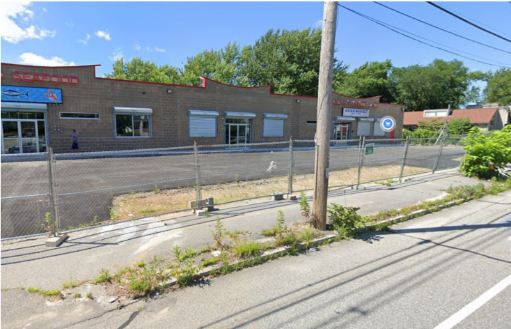
View of the building from Reservoir Ave
