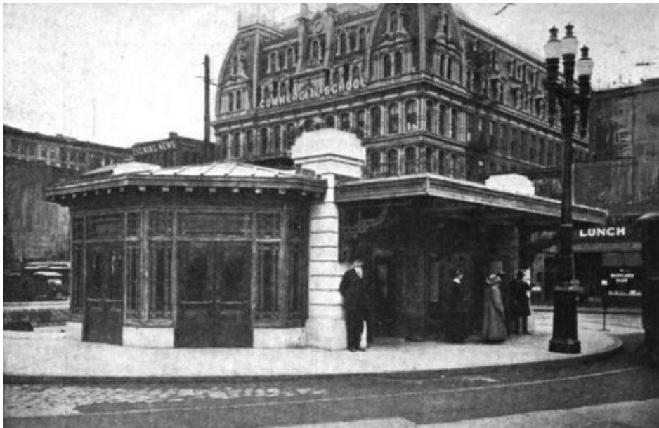
Trolley Shelter (and Public Comfort Station), c.1920 (RIHS)
