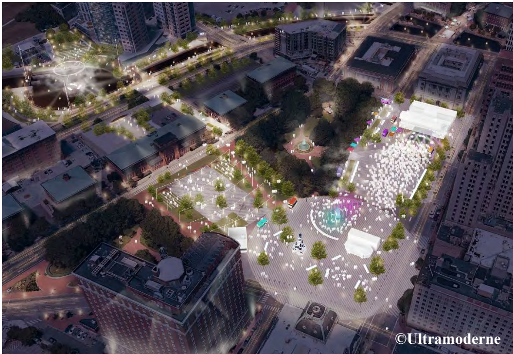
Photo 1 - Aerial View of Project
