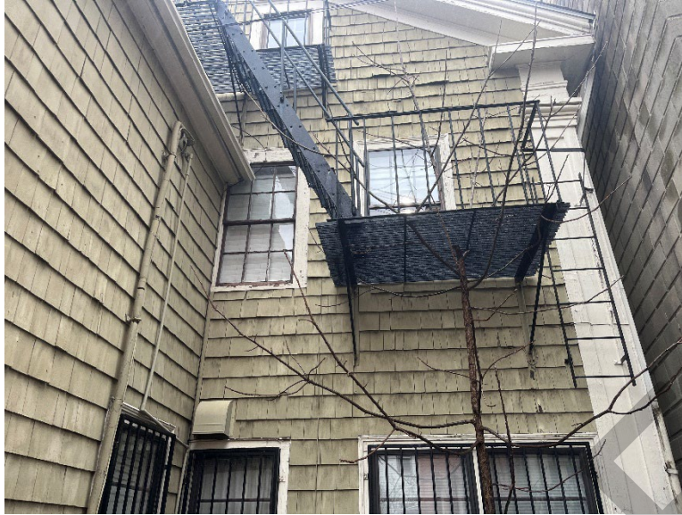
Figure 5 - detail view from south
