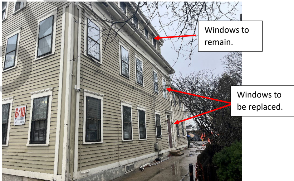
Figure 2 - Side view west
