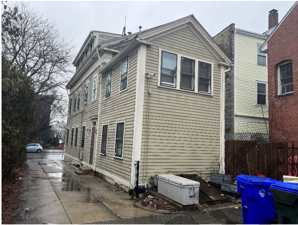
Figure 3 - view from back (south)
