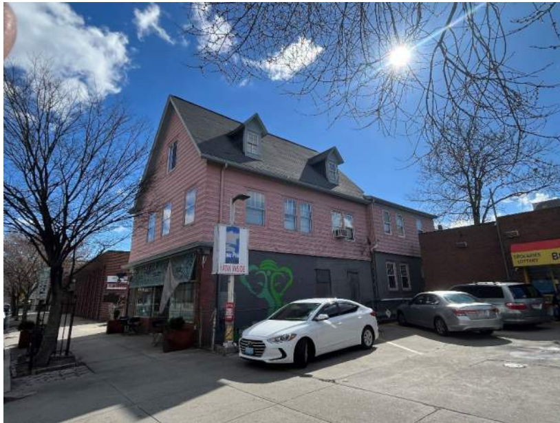
Figure 2 - View from NW corner
