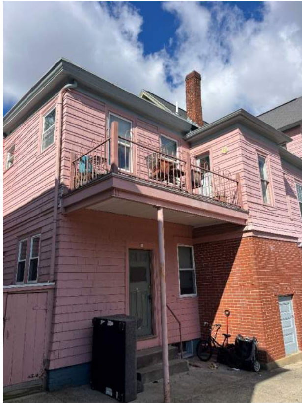
Figure 7 - view from SE corner
