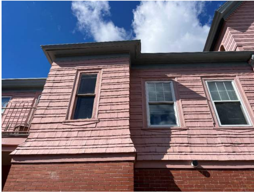
Figure 5 - detail at east wall
