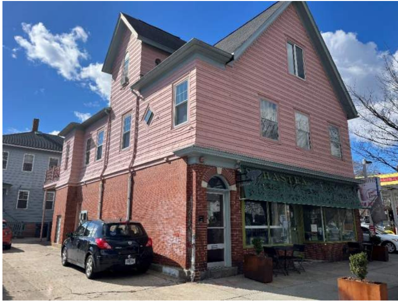
Figure 1 - View from NE corner
