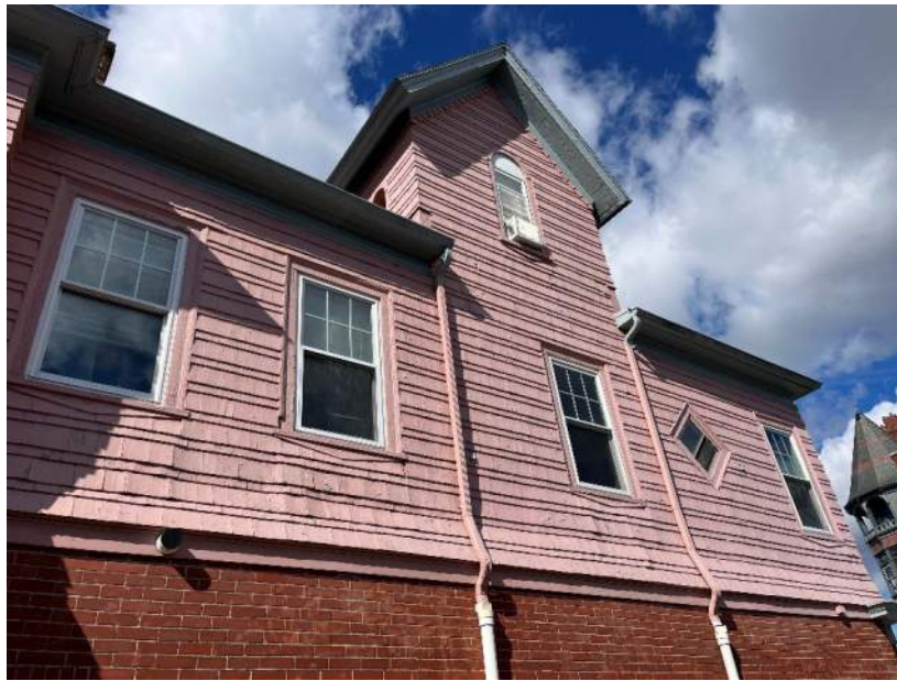
Figure 4 - view of east wall
