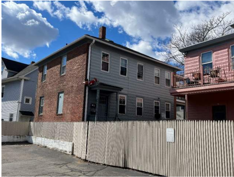
Figure 1 - View from NE corner
