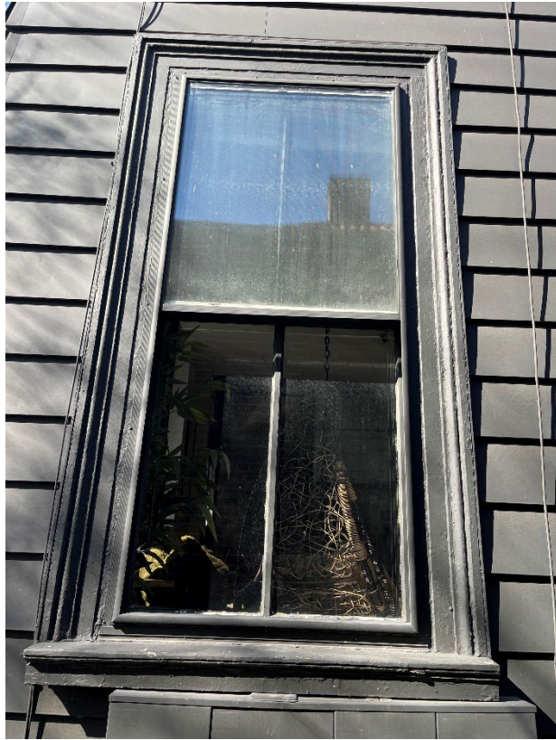
Figure 6 - Unit "B" - wood, single glazed w/ storm window
