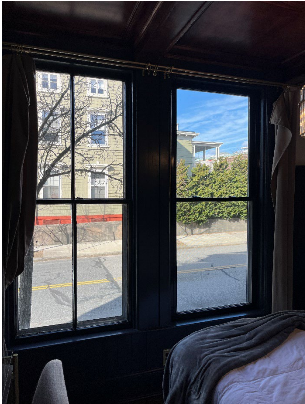
Figure 14 - interior at unit's "B" & "C"
