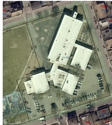
Aerial view of the site
