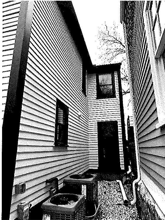
Figure 6 - Partial NW corner
