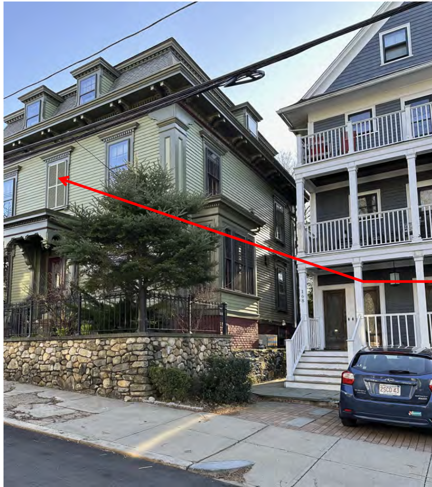
Figure 2 - Northeast Corner, Viewed from Prospect St.
