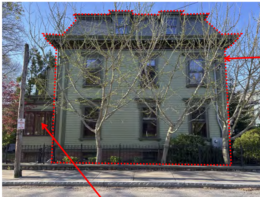
Figure 3 - South Facade, Viewed from Hidden St.
