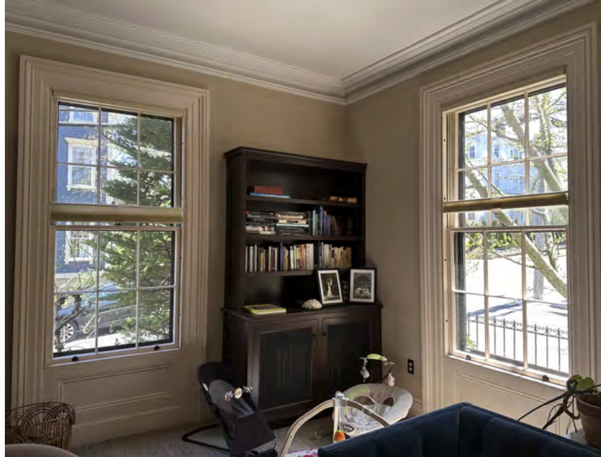
Figure 8 - Typical interior condition at first floor
