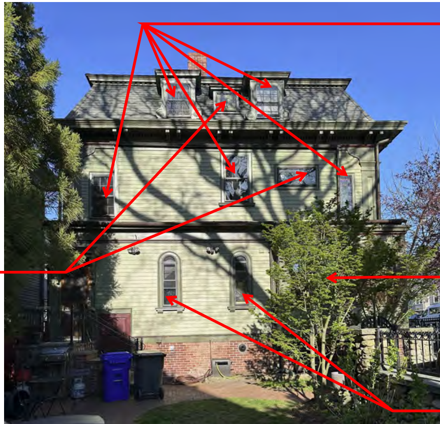
Figure 5 - West Facade, Viewed from Yard
