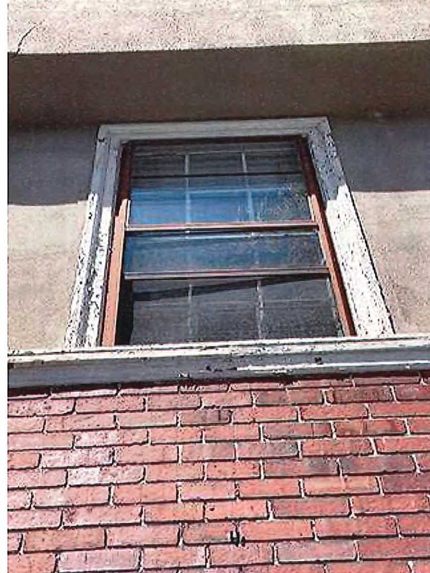
EXISTING WINDOW INSTALLATION AT STUCCO SHOWING EXTERIOR MOUNTED ATORM WINDOWS
