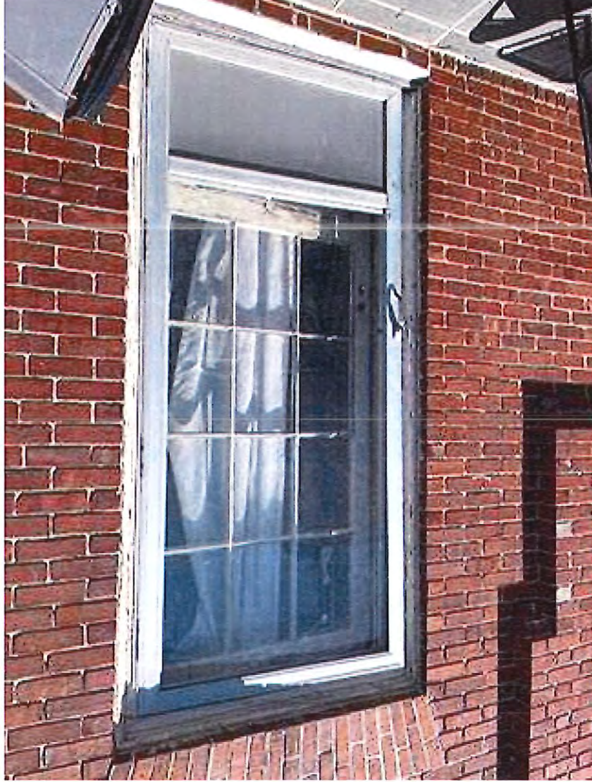
EXISTING SOUTHWEST CORNER EXTERIOR TERRACE DOOR
