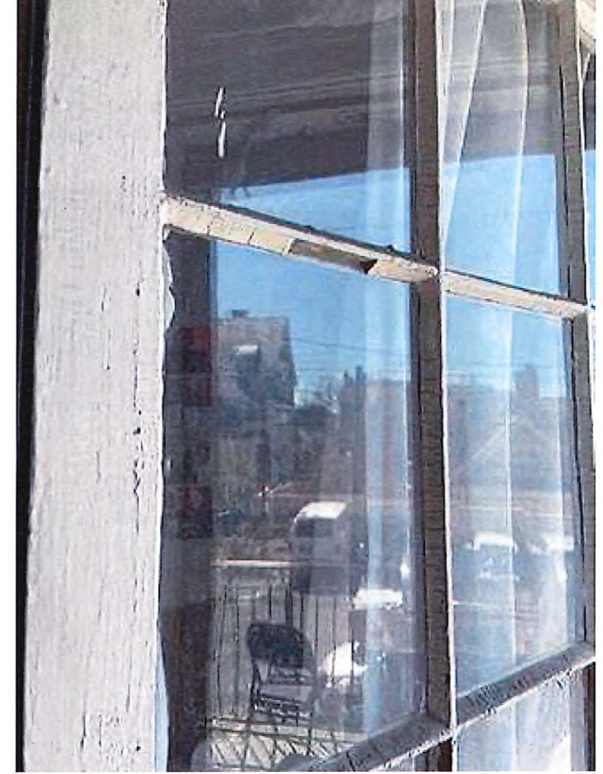
EXISTING EXTERIOR TERRACE DOOR GLASS LITES & MUNTINS
