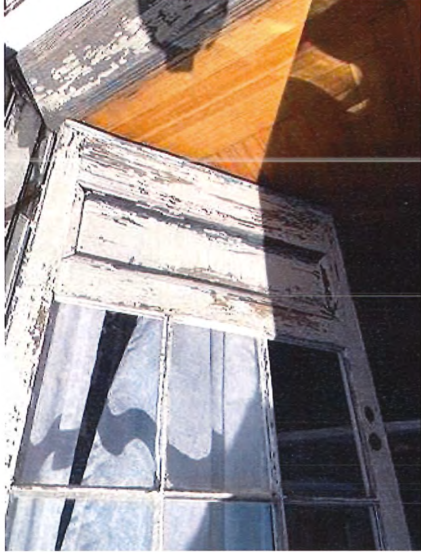
EXISTING EXTERIOR TERRACE DOOR
