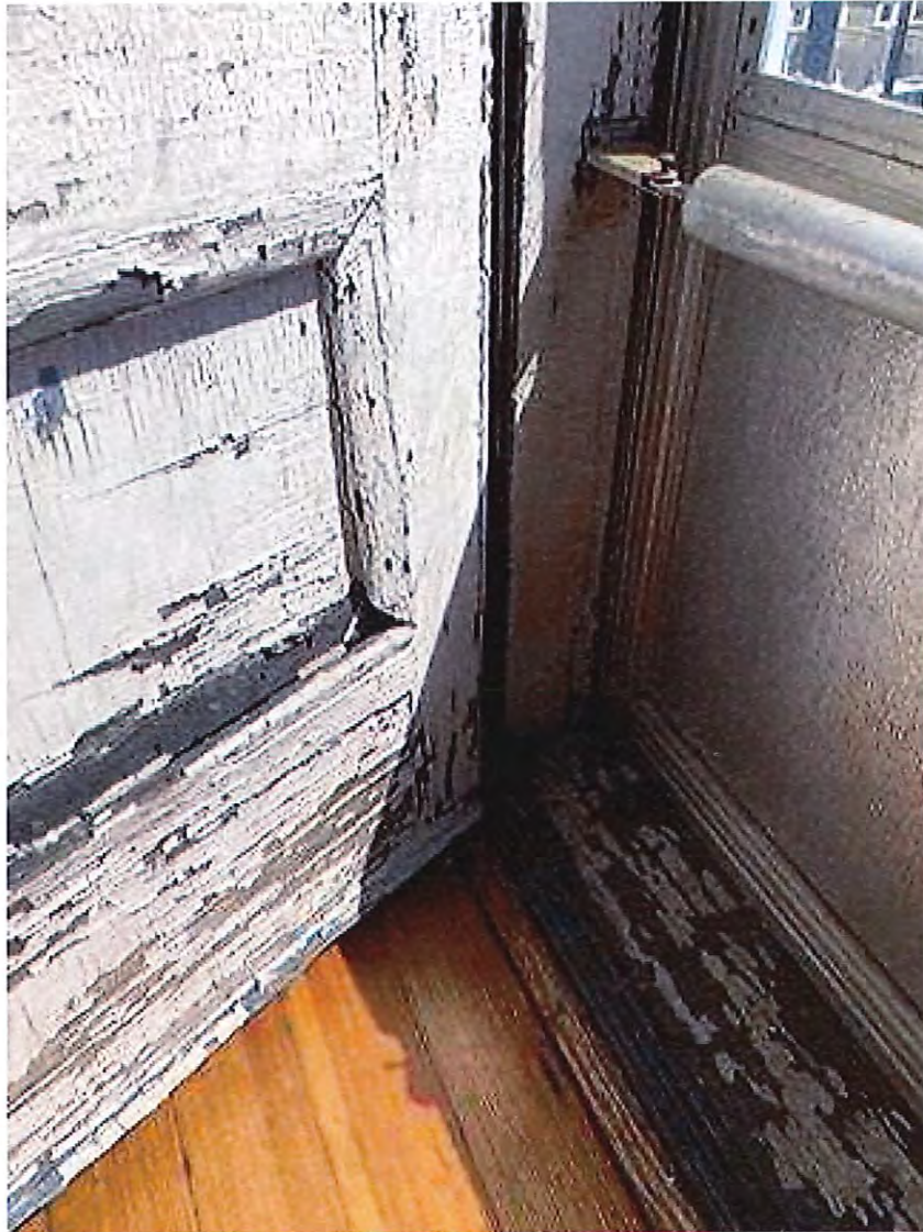
EXISTING EXTERIOR TERRACE DOOR RECESSED PANEL, SILL & JAMB
