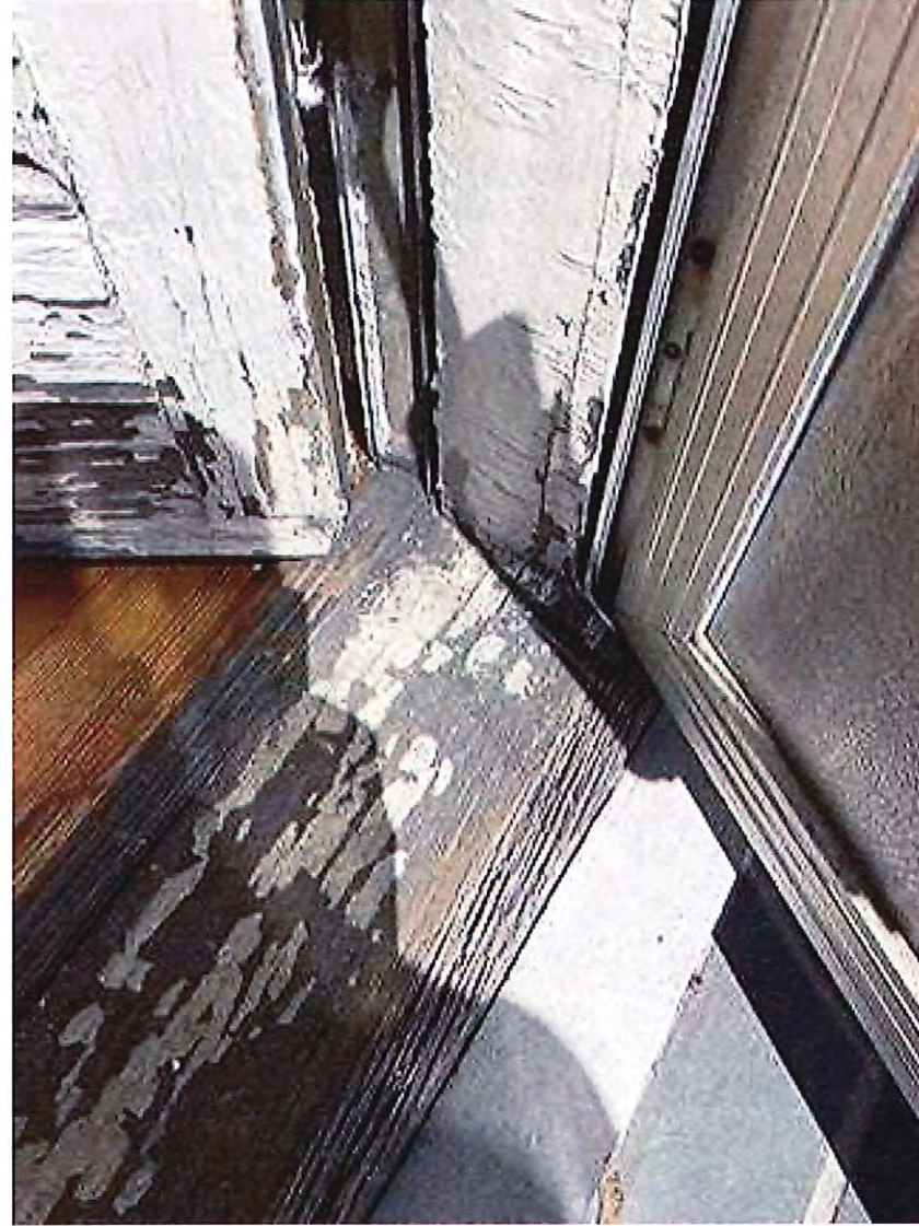
EXISTING EXTERIOR TERRACE DOOR WOOD SILL & JAMB
