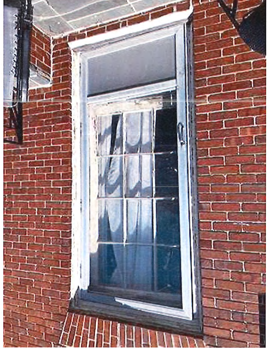
EXISTING SOUTHEAST CORNER EXTERIOR TERRACE DOOR
