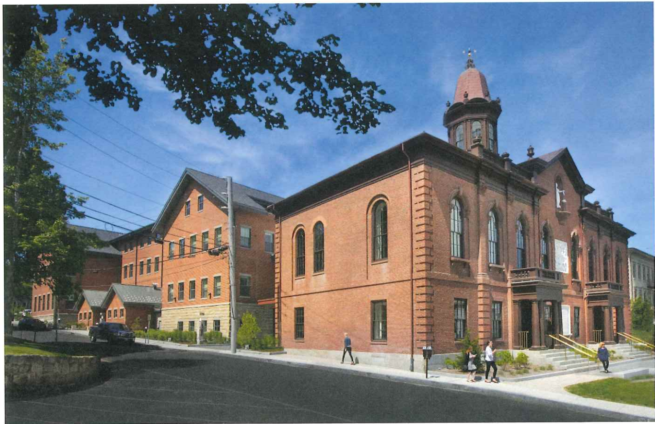
Project: Plymouth Town Hall Location: Plymouth, MA Size: 76,048 sf Completion Date: 2017 Construction Cost: $30M Client: Town of Plymouth Client Contact: Melissa Grabau Arrighi, Former Town Manager, 508.889.5683
