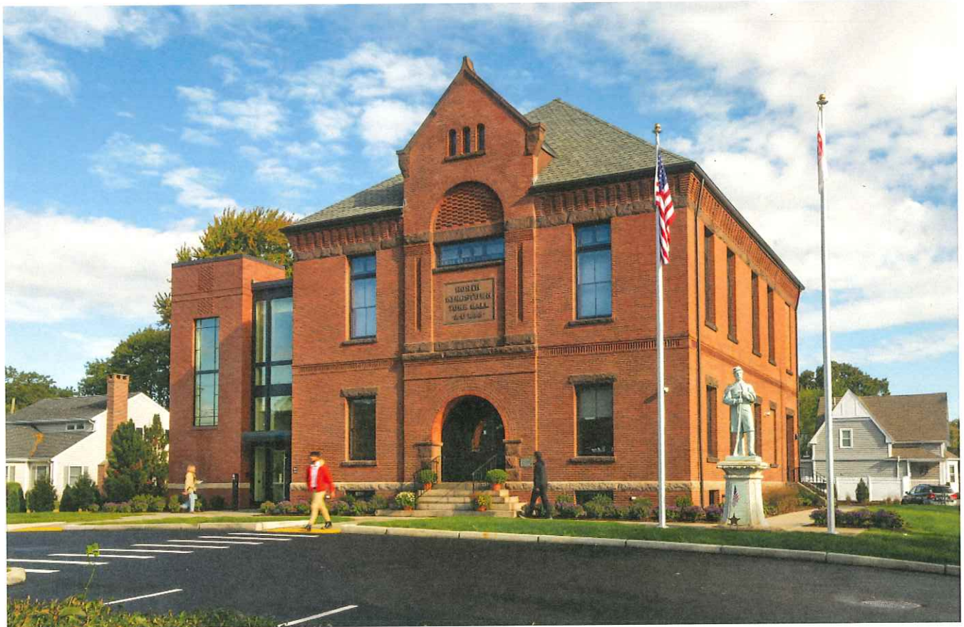
Project: North Kingstown Town Hall Location: North Kingstown, RI Size: 7,400 sf Completion Date: 2022 Client: Town of North Kingstown Client Contact: Ralph Mollis, Town Manager, RMollis@northkingstown.org, 401.268.1501
