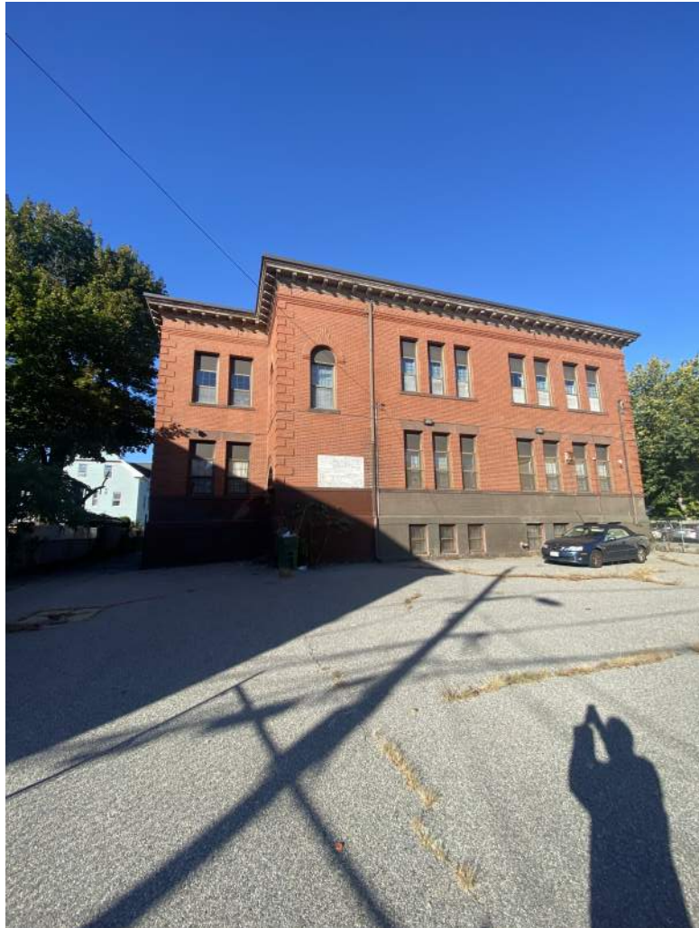
Photograph – 1: Photo depicts the structure as scheduled for planned renovation.
