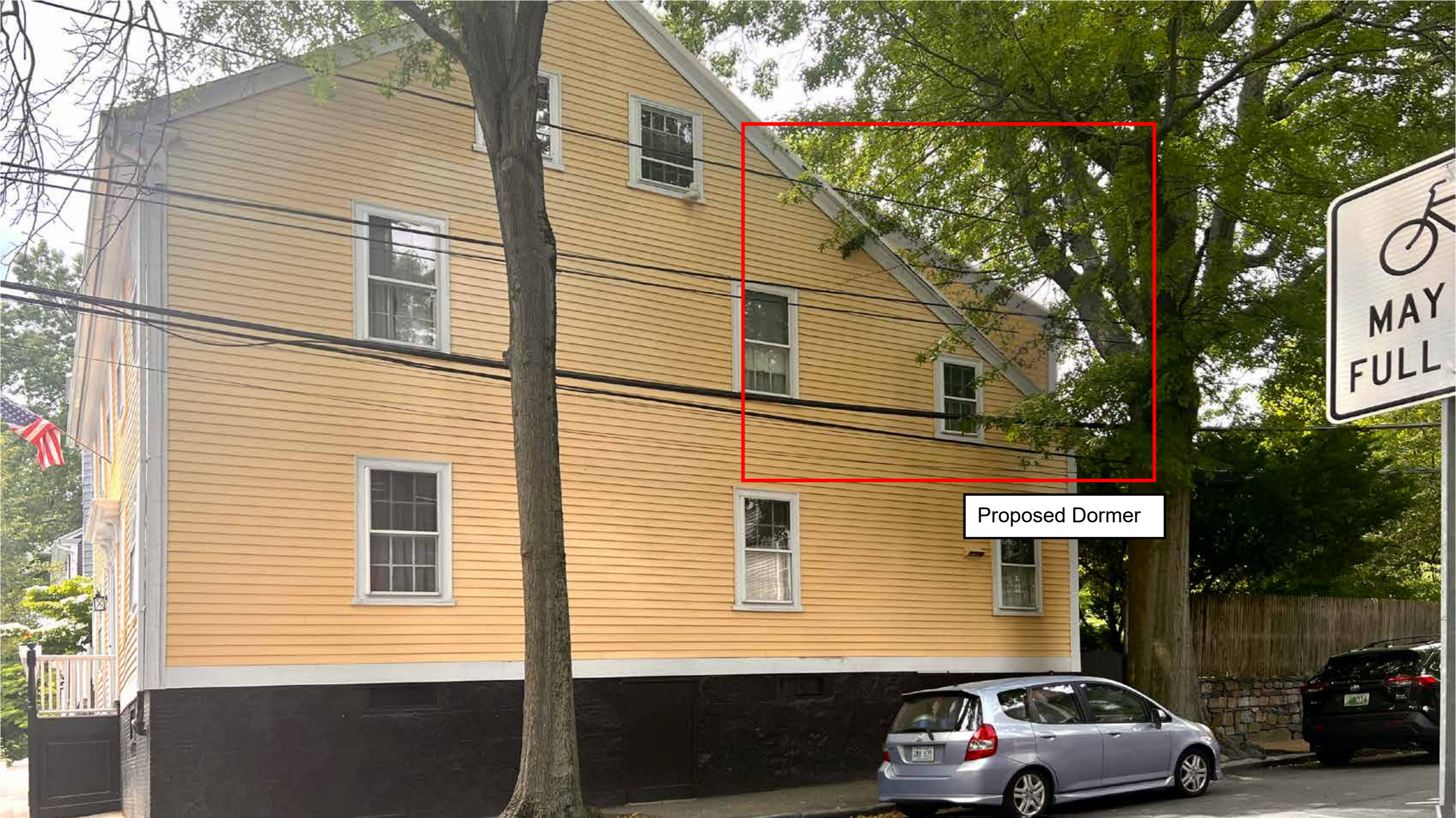
Proposed dormer viewed from the intersection of Thayer Street and John Street
