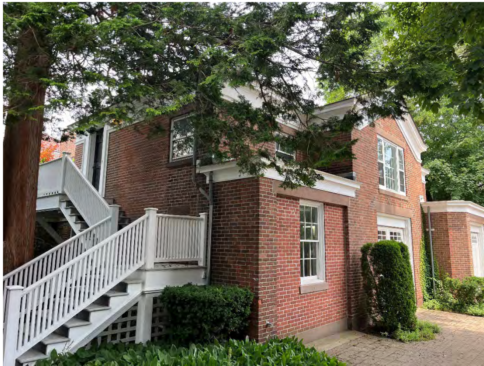
Figure 12 - Carriage House NW corner
