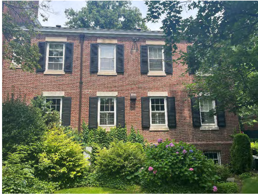
Figure 7 - portion of south wall
