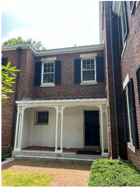
Figure 4 - secondary entry - north
