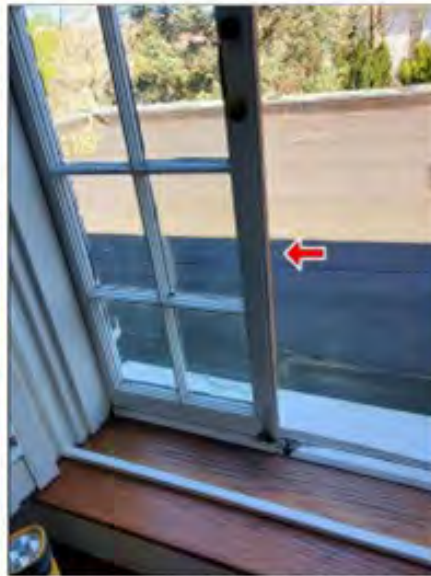
7.0 INTERIOR WINDOWS (Picture 8)
