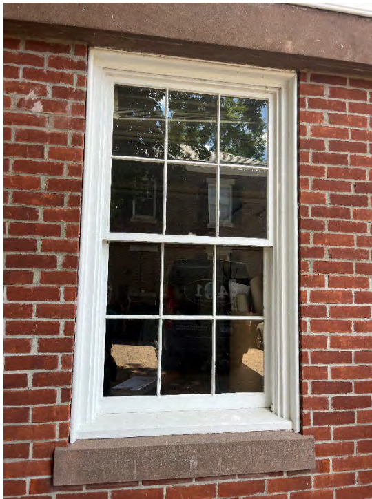
Figure 16 - Carriage House unit "K"
