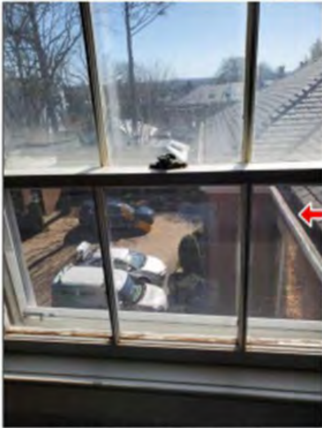
7.0 INTERIOR WINDOWS (Picture 10) 3rd fl left side.
