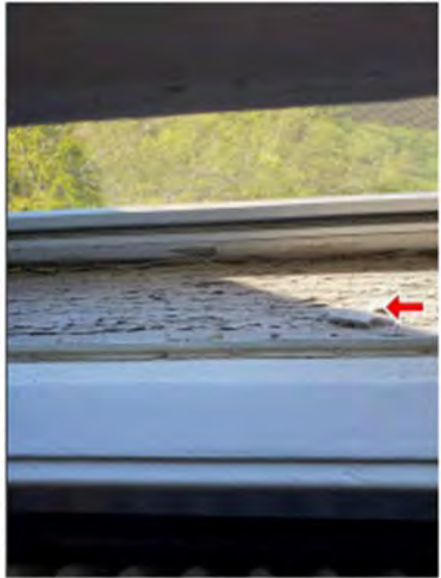
7.0 INTERIOR WINDOWS (Picture 11)
