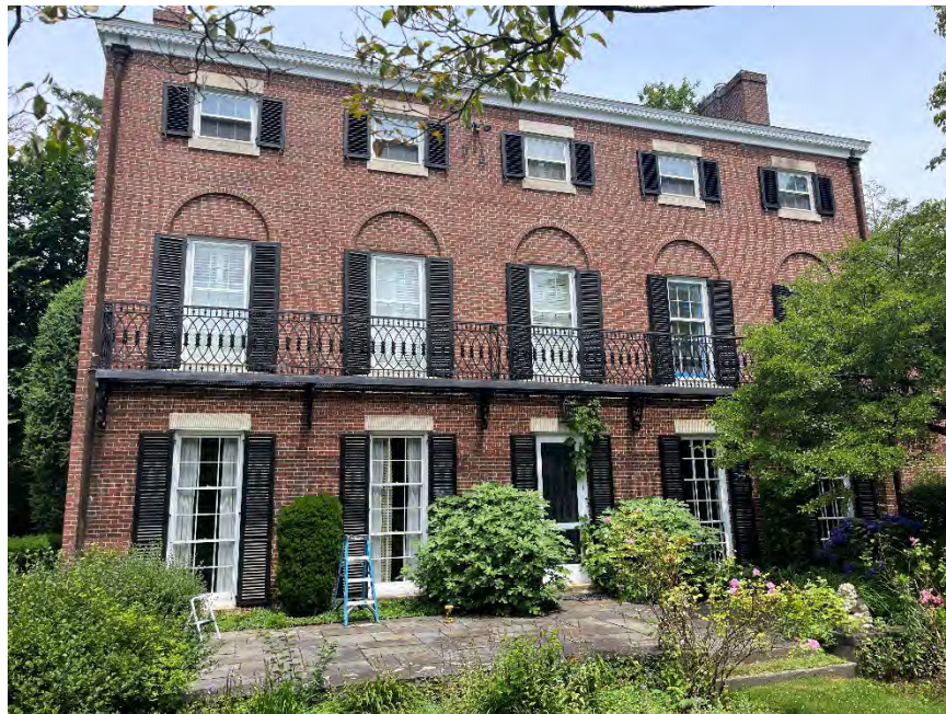
Figure 8 - portion of south wall
