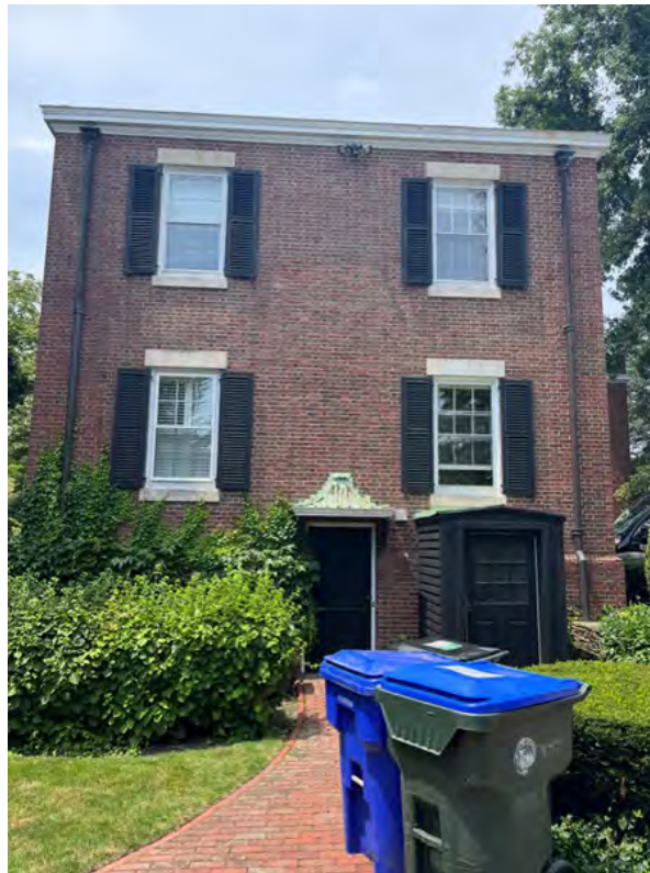
Figure 6 - end of east wing
