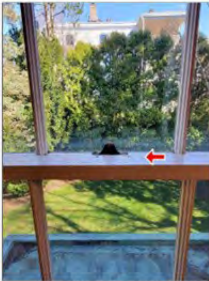
7.0 INTERIOR WINDOWS (Picture 7)
