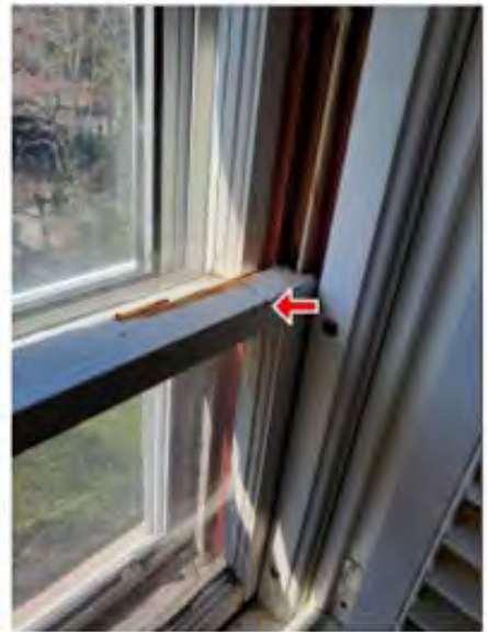
7.0 INTERIOR WINDOWS (Picture 9)
