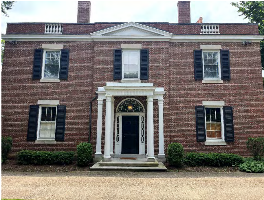
Figure 1 - North wall - Entry
