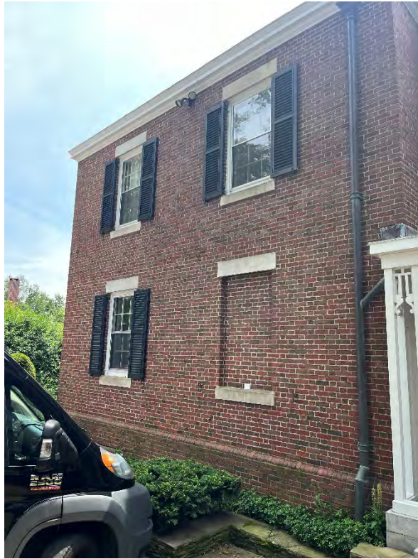
Figure 5 - portion of north wall
