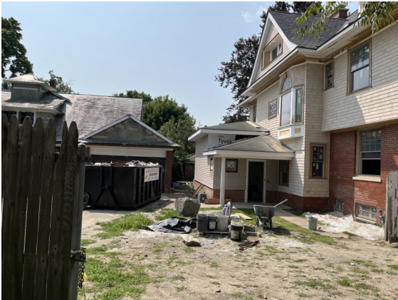
View of the lot from Wayland Ave
