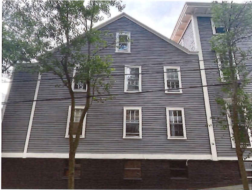
Figure 3 - view 2 from Arnold Street
