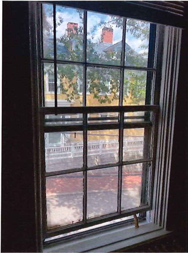
Figure 9 - Interior unit "B"
