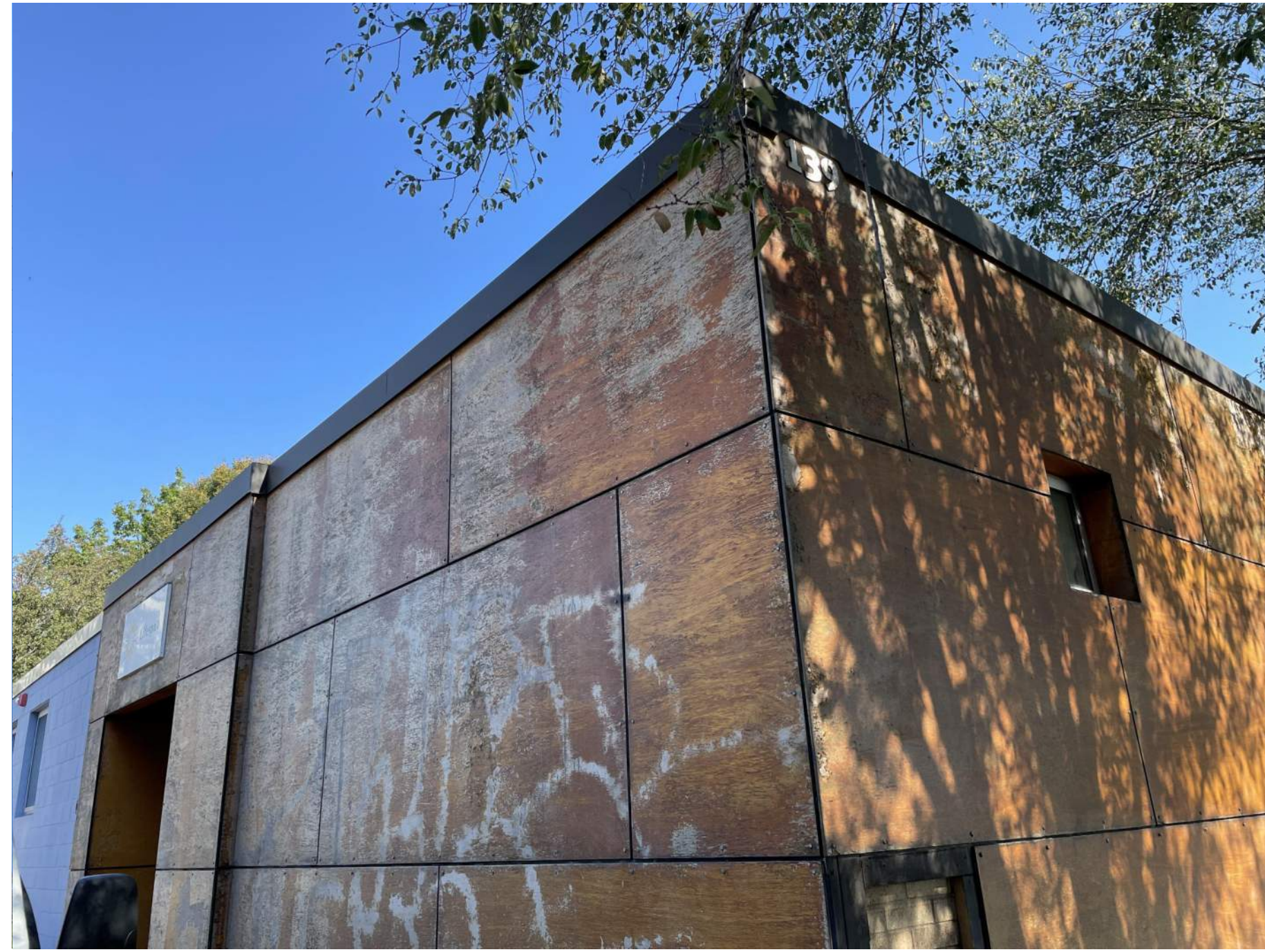
EXISTING PHOTO A
