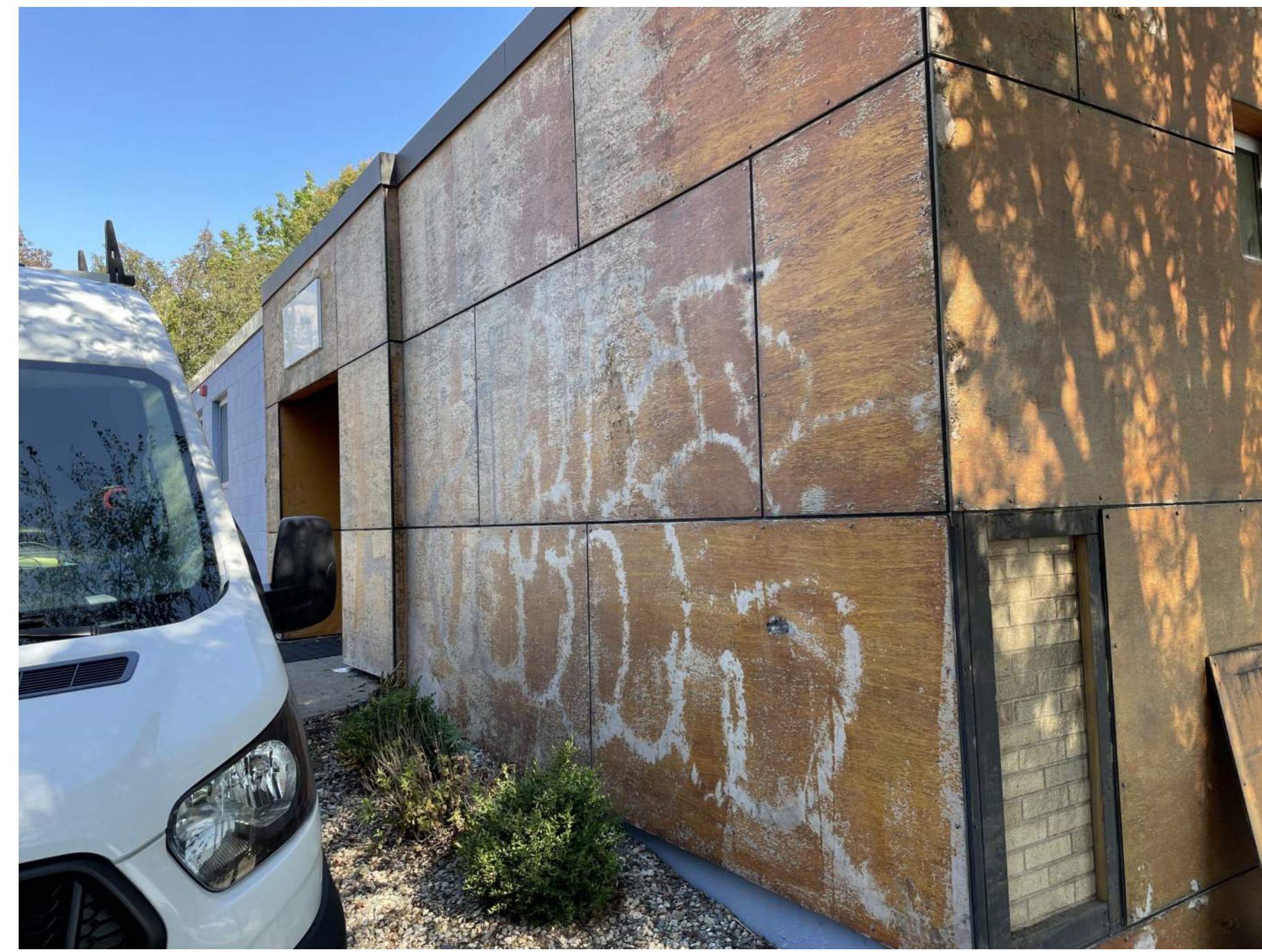
EXISTING PHOTO B
