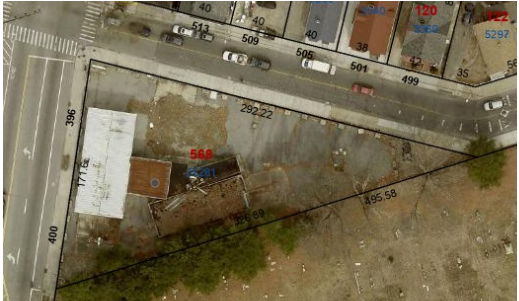
Aerial view of the site
