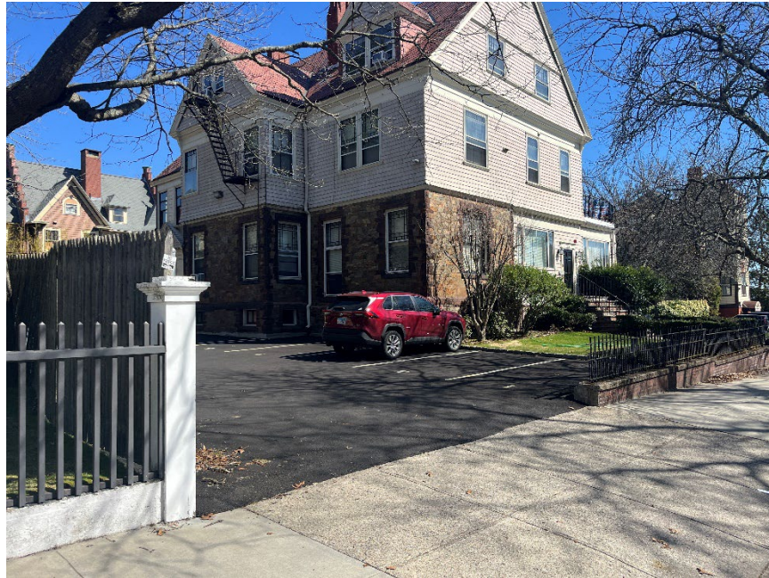
Figure 4 - main house SW corner
