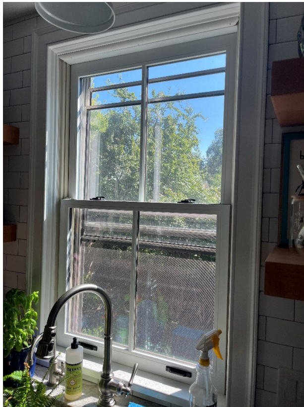
Figure 18 - Interior window "D" - Trimline unit
