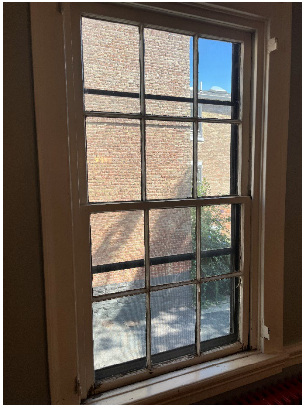
Figure 14 - Interior at window "A"
