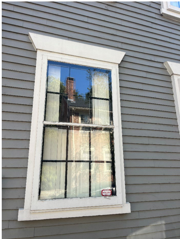
Figure 10 - Window "A" on street
