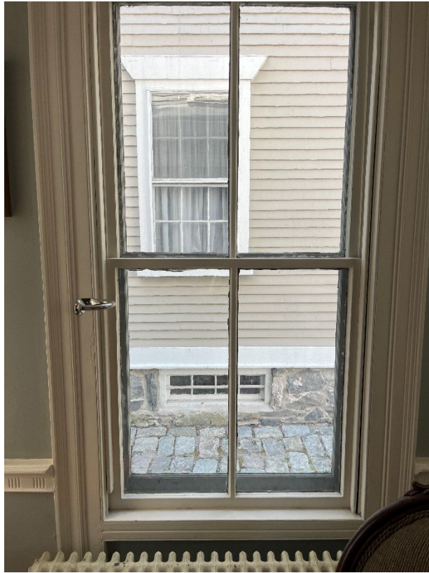
Figure 17 - Interior window "C"
