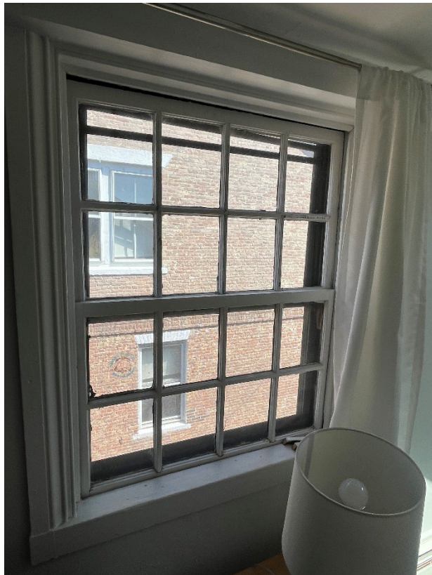
Figure 24 - Interior window "G"
