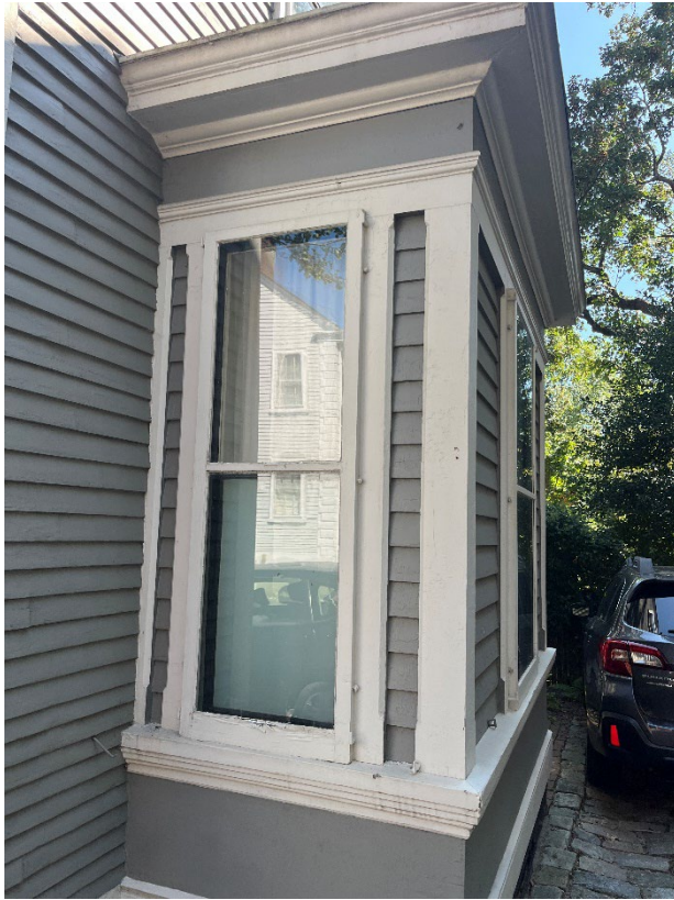
Figure 11 - Window "B" facing street
