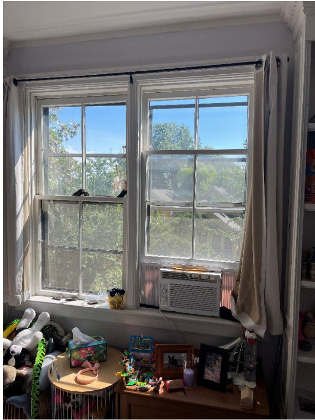
Figure 23 - Interior windows "F"
