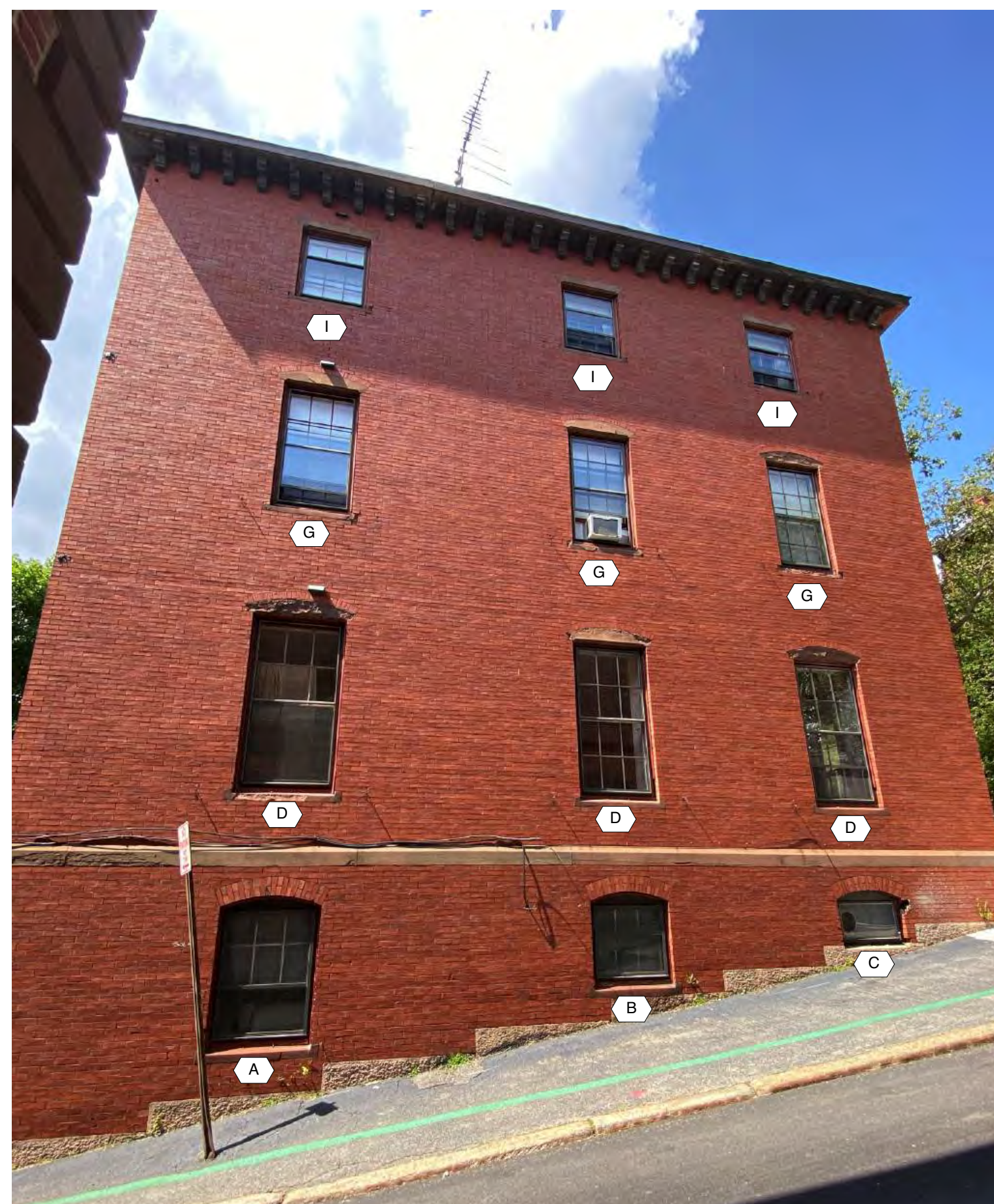
3 DD.4 SOUTH ELEVATION (LOOKING NORTH FROM N COURT ST)
