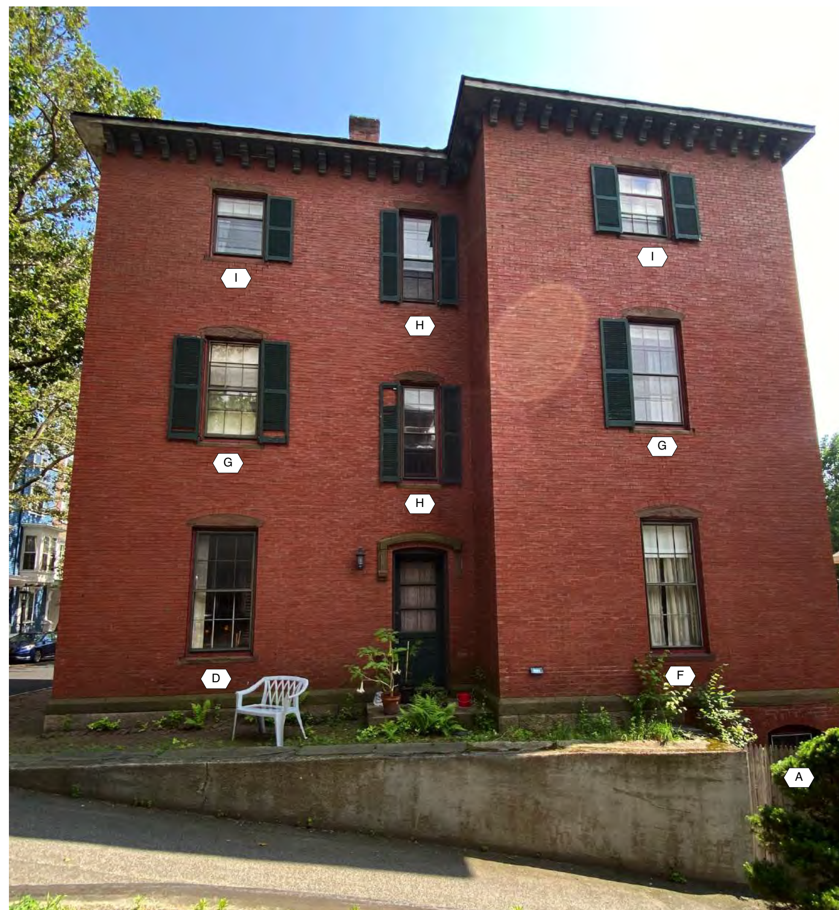
3 DD.3 NORTH ELEVATION (LOOKING SOUTH FROM ADJACENT LOT)
