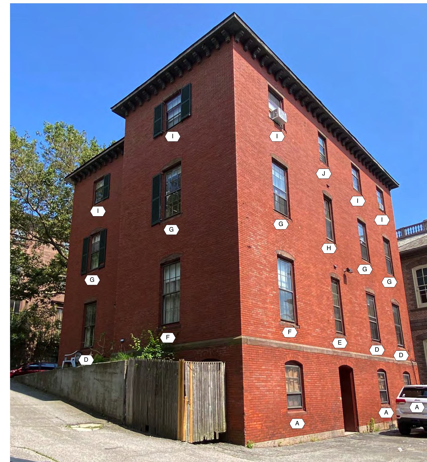
4 DD.3 NORTH WEST CORNER (LOOKING SOUTH EAST FROM PARKING LOT)
