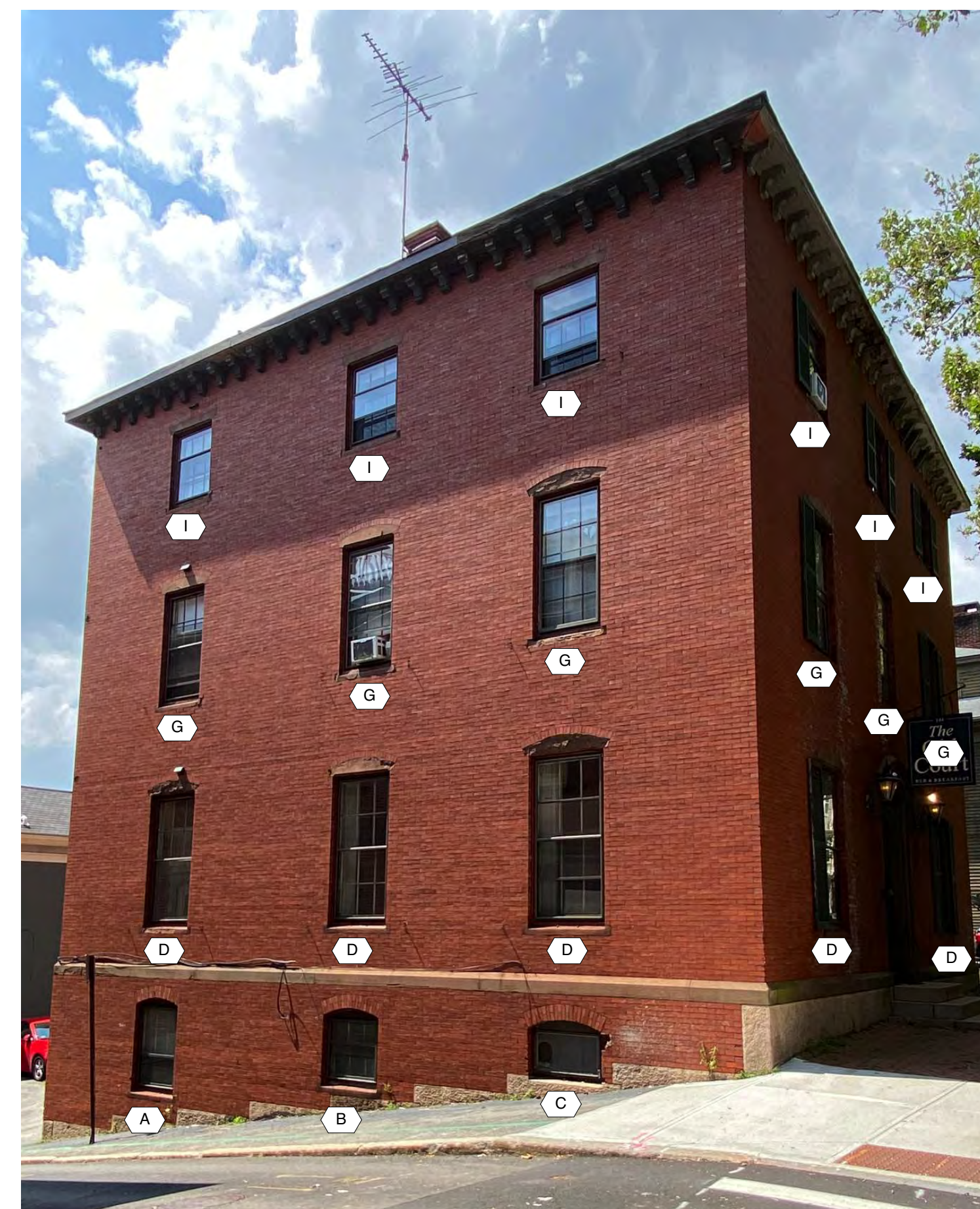
4 DD.4 SOUTH EAST CORNER (LOOKING NORTH FROM N COURT ST)
