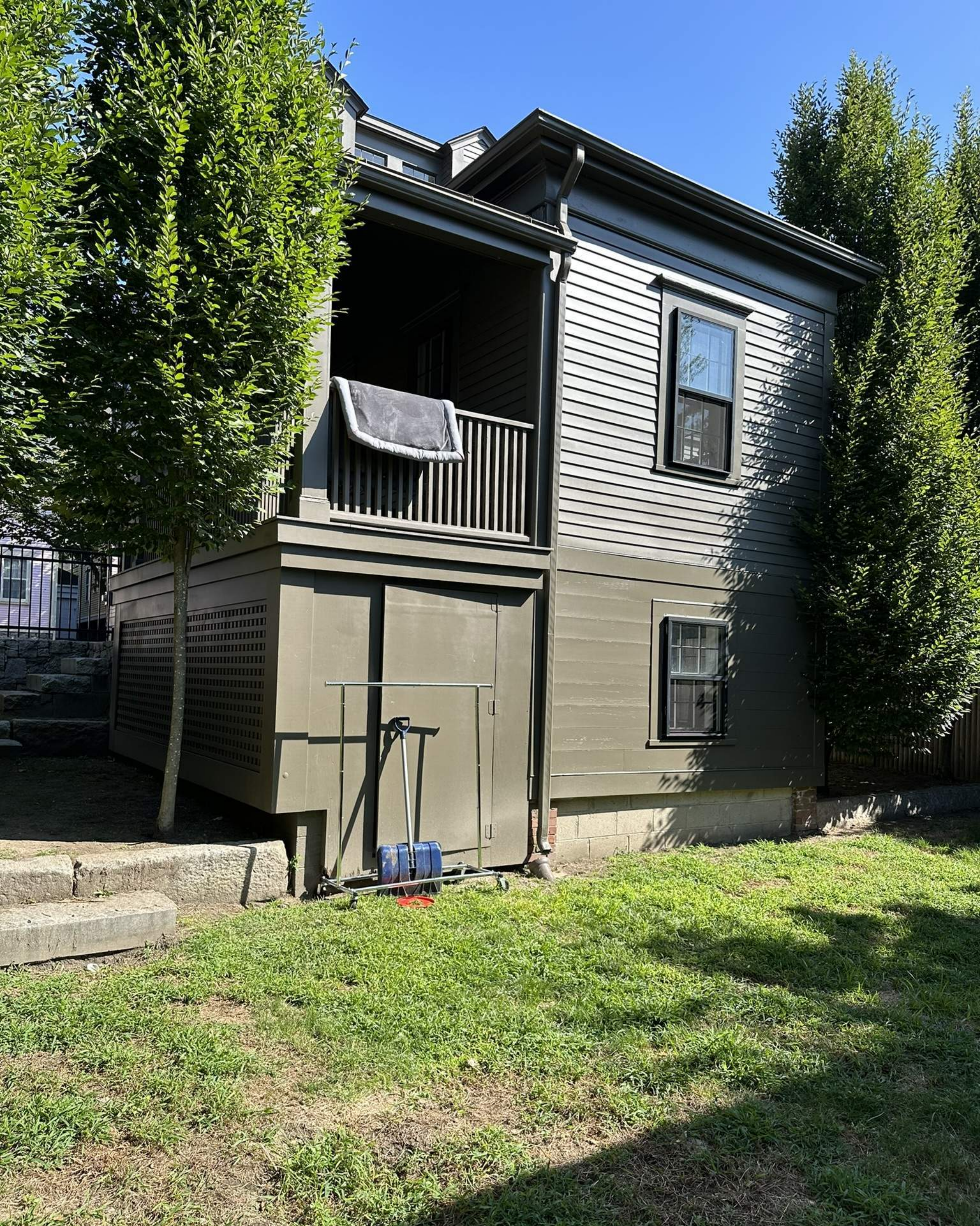
View 6 - South elevation of rear ell with attached side entry porch.
