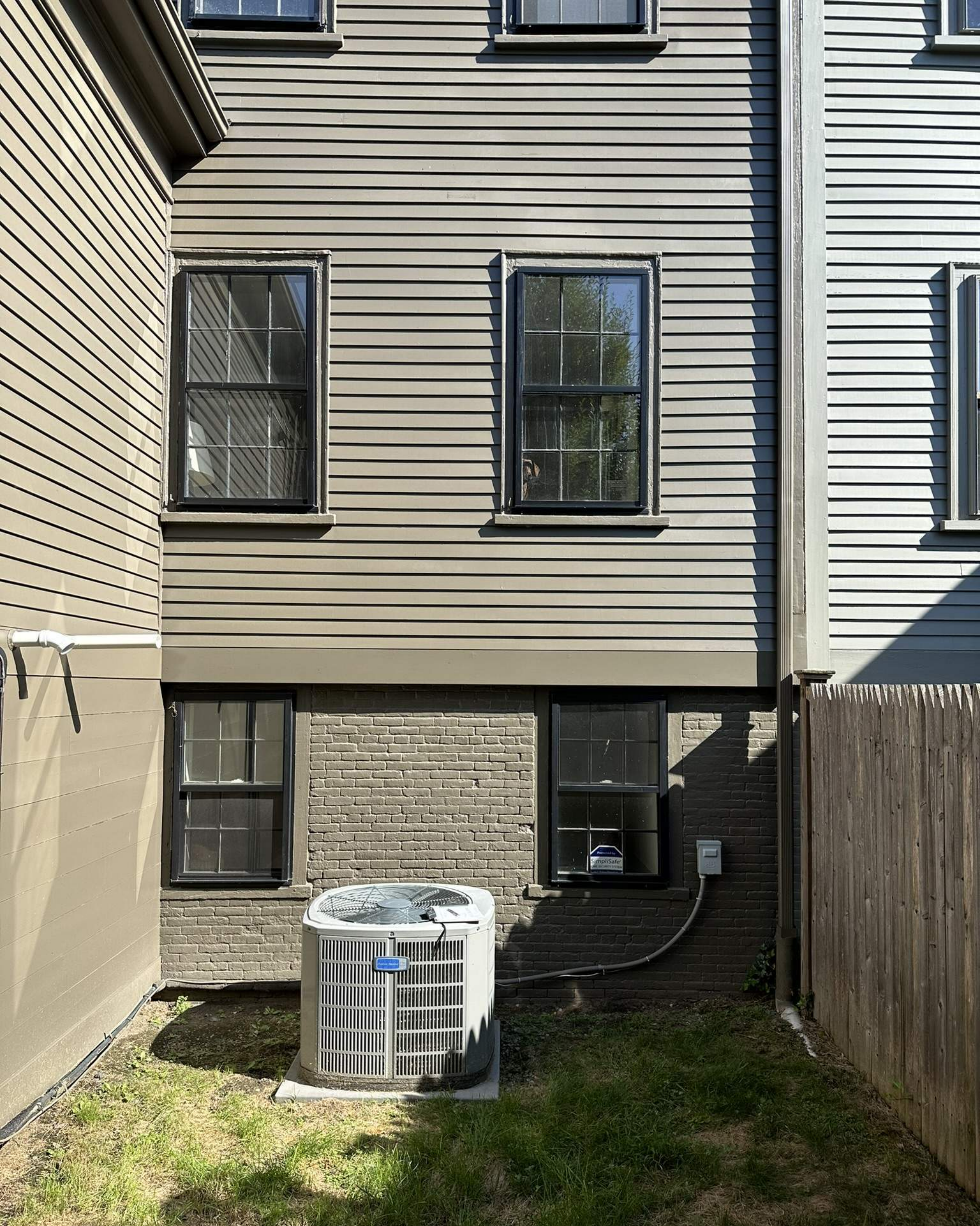
View 10 - Courtyard to east of rear ell addition.
