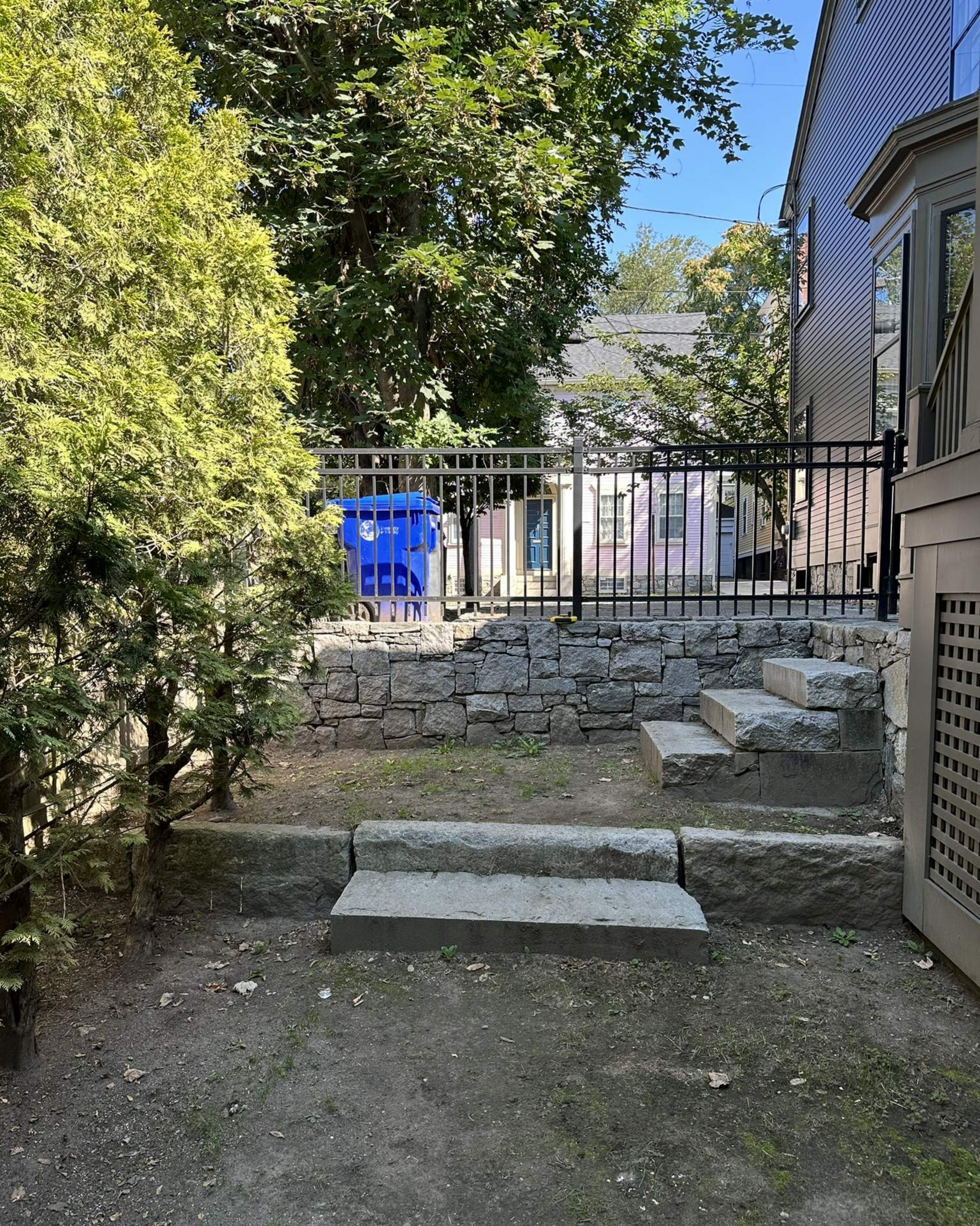
View 5 - Rear yard access - looking to north towards driveway.
