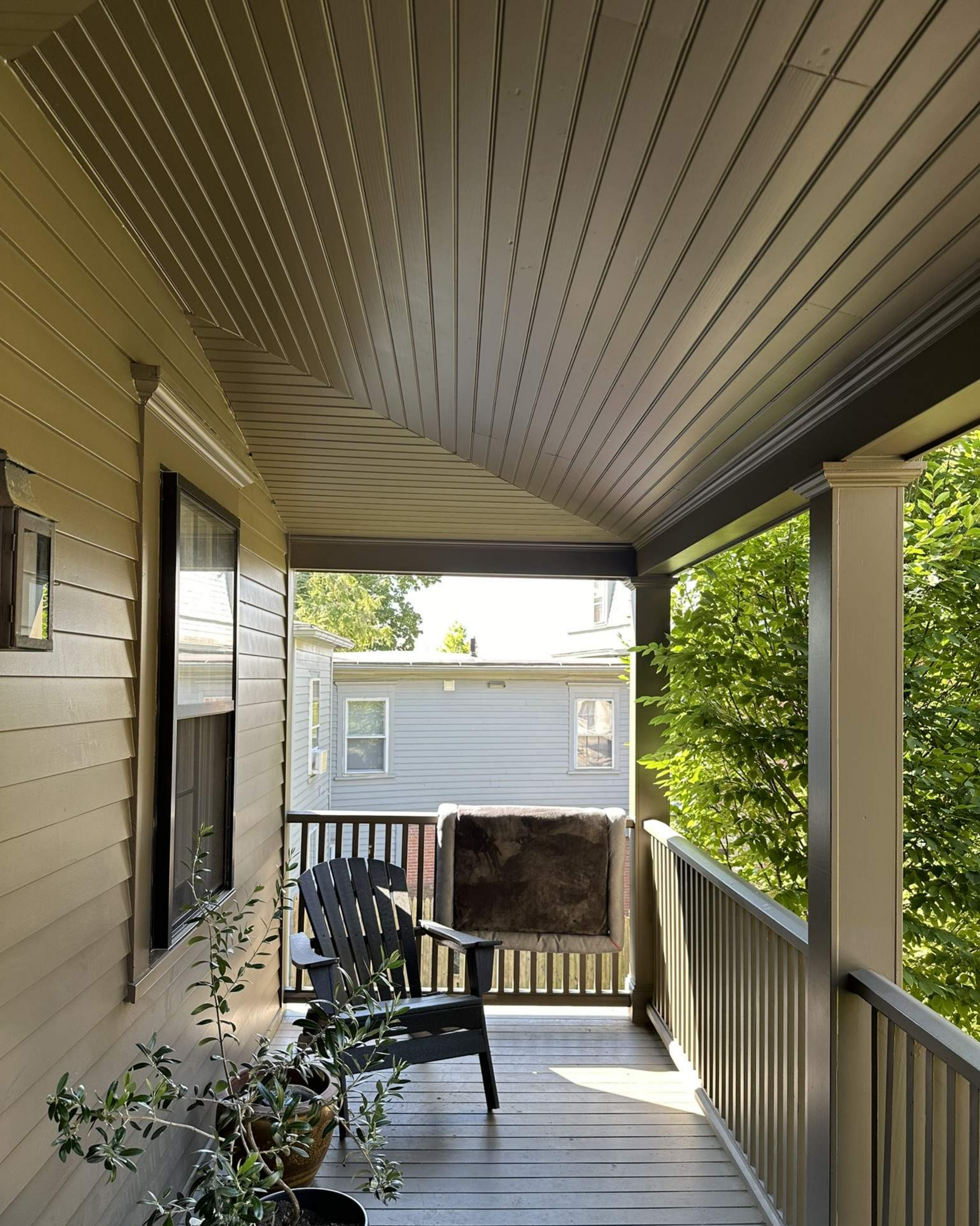
View 4 - Side entry porch of rear ell addition.
