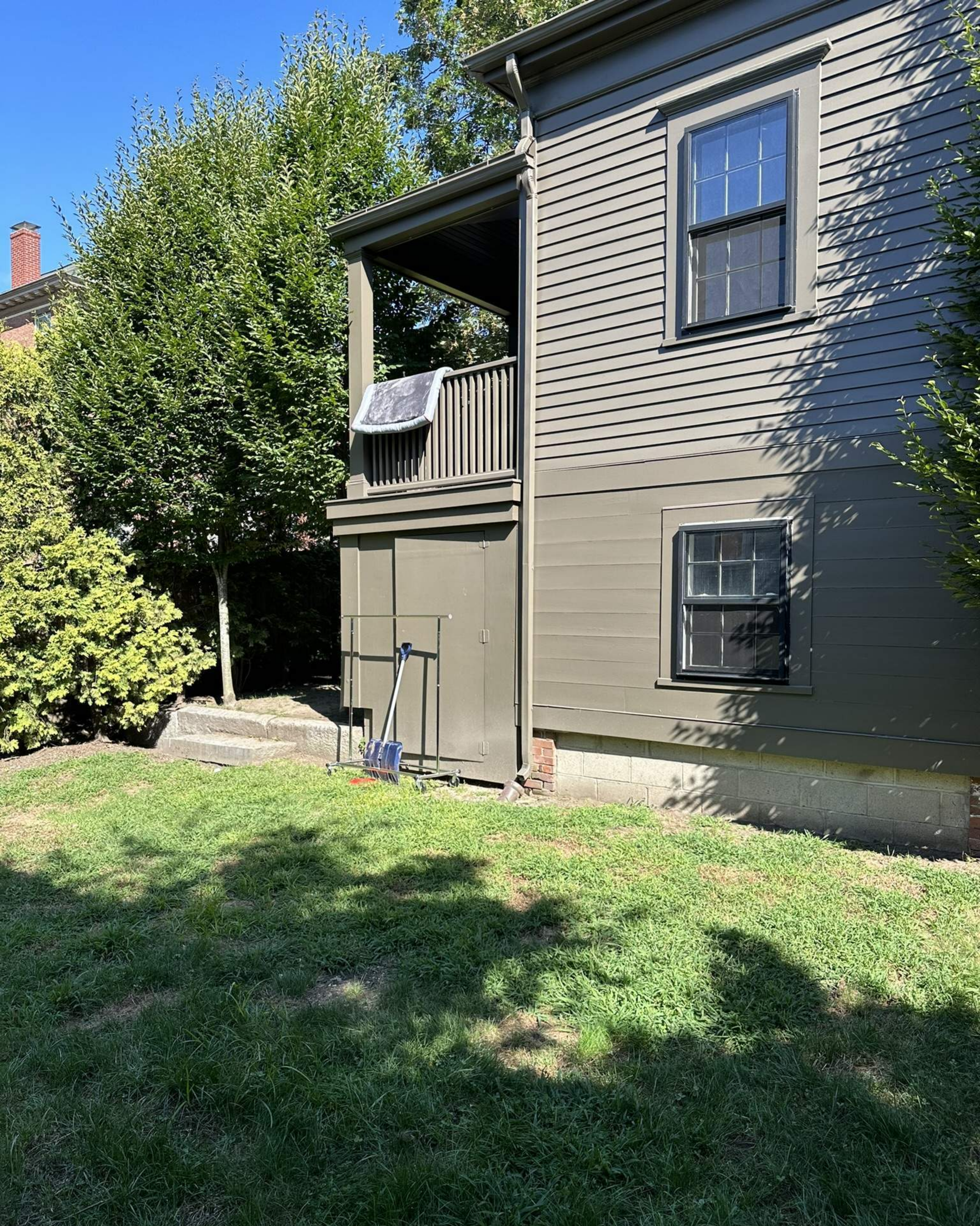
View 7 - South elevation of rear ell with attached side entry porch.
