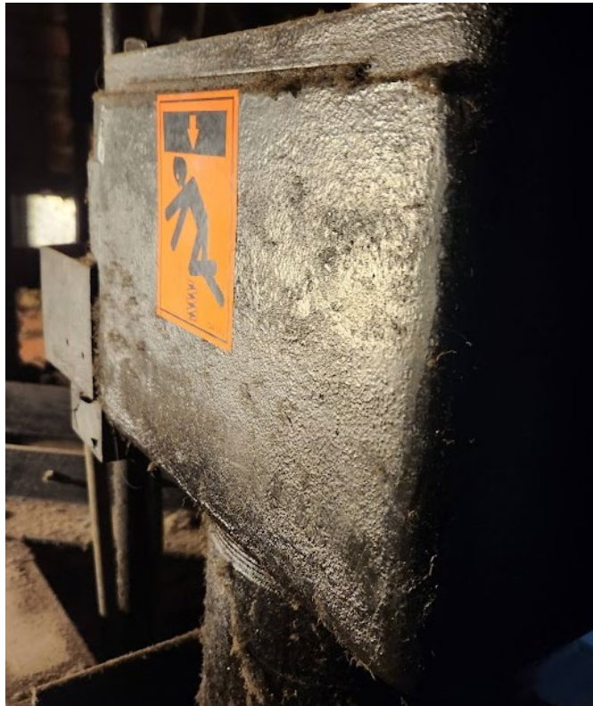
Potential PCB containing oil reservoir example.
