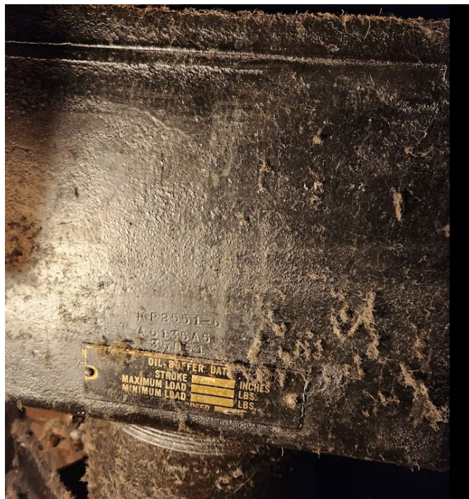
Potential PCB containing oil reservoir example.
