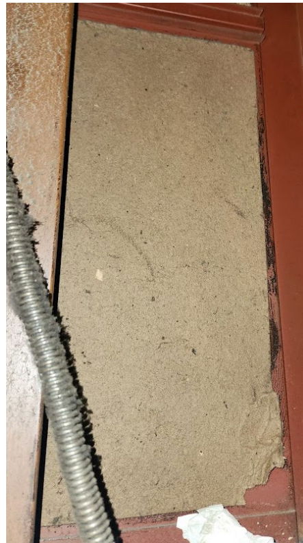
Masonite paneling at interior shaft. Paneling and glue negative for asbestos.
