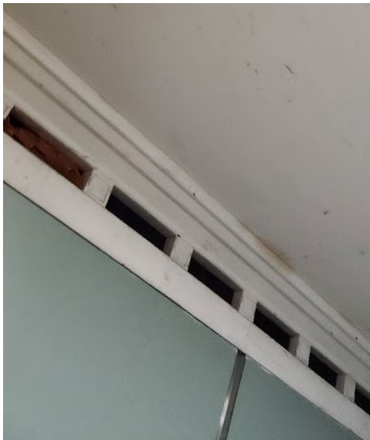
Interior carriage paint non-LBP.
